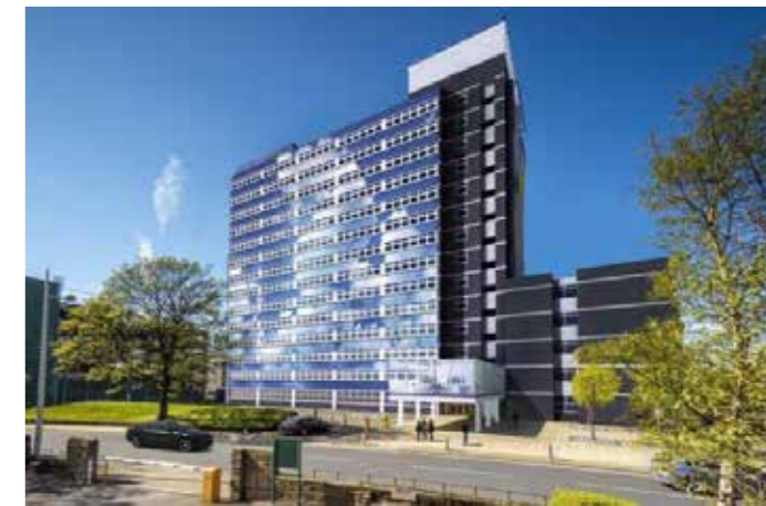
Daniel House Residential Conversion
